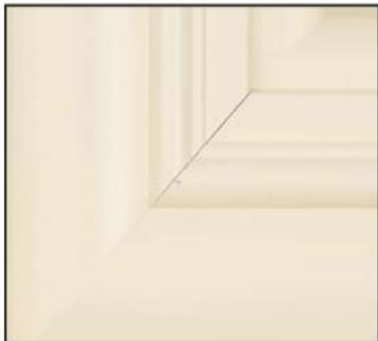
Example of door front joint separation
